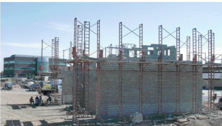
Block overruns were used in this project to save construction material costs.
